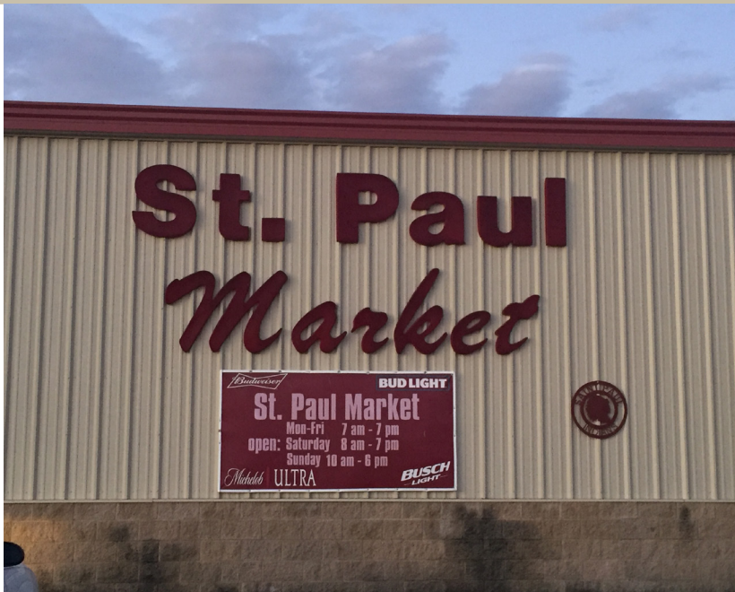
The St. Paul Supermarket sits along highway 47 in St. Paul, Kansas.
